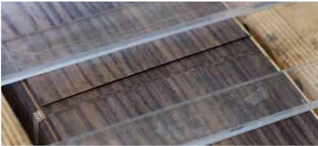
Remove the wood between the scored lines with a router or chisel, just deep enough for the thickness of the end trim.
